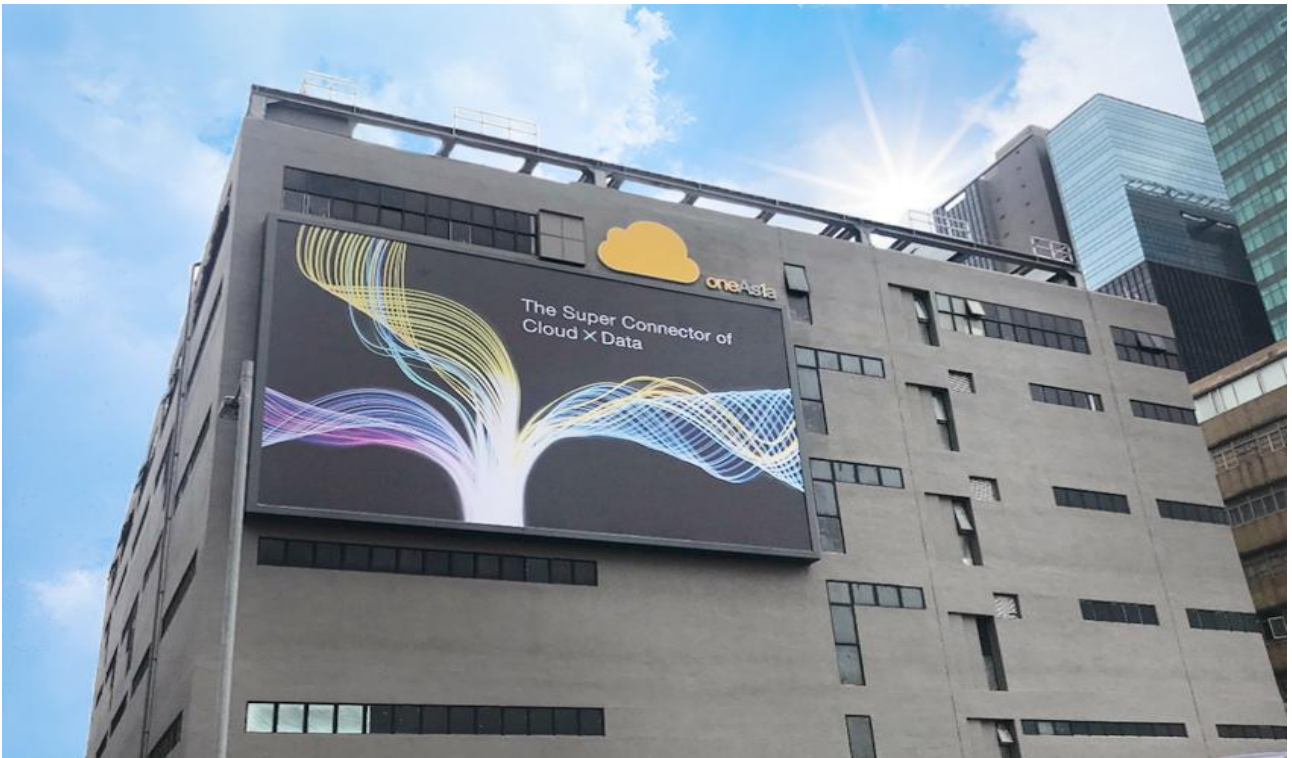
OneAsia Kowloon Bay Data Center
